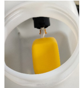
Picture 6.b Float valve in-side tank
